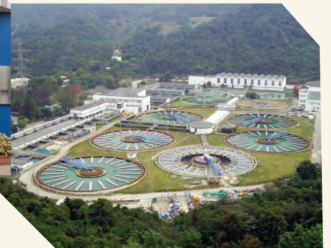
Water Treatment Works
