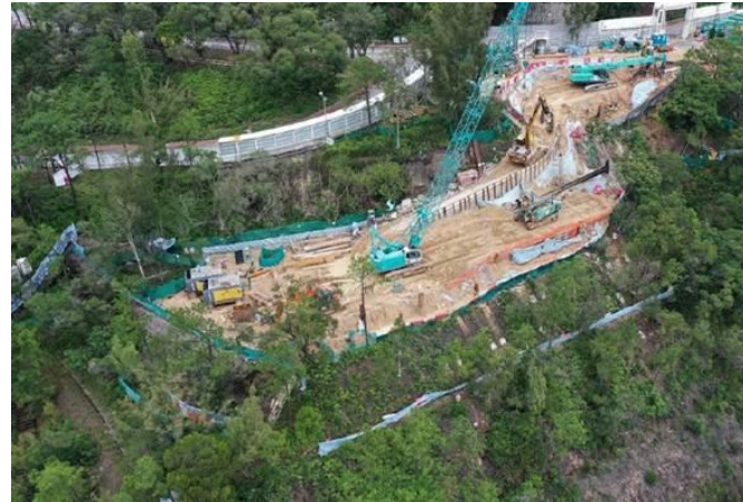
Piling Works at Lower Platform – Block 1&2
