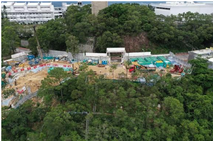
Piling Works at Upper Platform – Block 3&4
